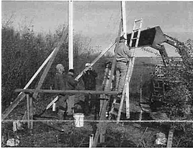
The work crew positions the uprights for the billboard sign.
